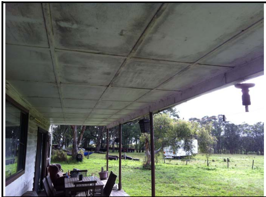
Photo 6: A section of the ACM sheeting used on the underside to the verandah on the back and southern side of the house
