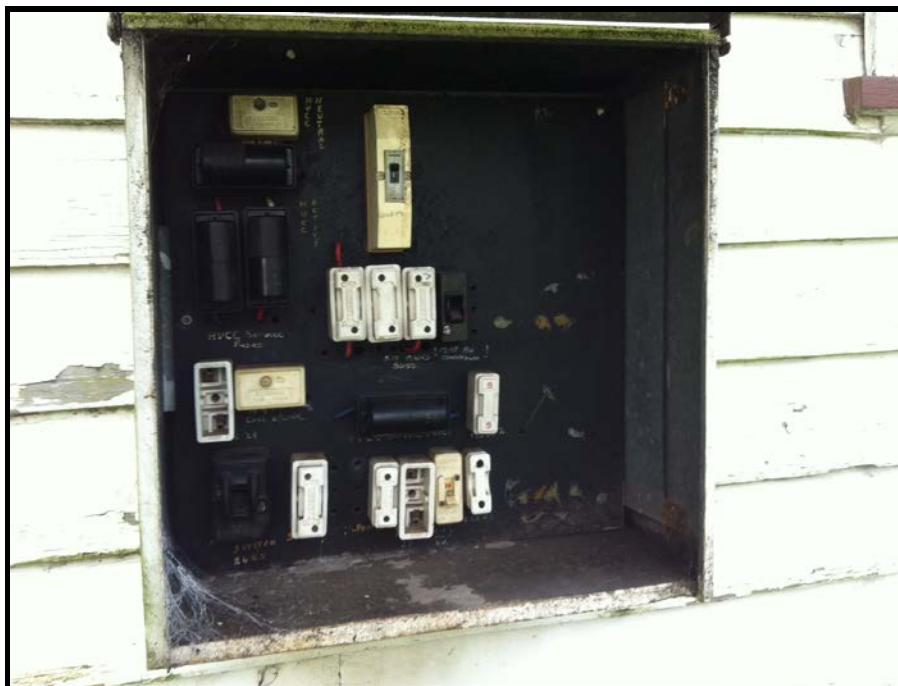
Photo 12: The electrical power box to the house with a zelemite backing board.
