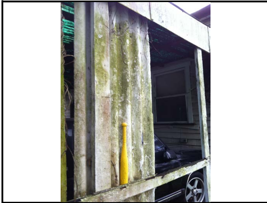
Photo 1: Part of the corrugated AC sheeting southern wall to the carport on the western side of the house (sheets on the northern side of the carport appeared to have been removed). Also note the ACM panelling above the corrugated sheeting
