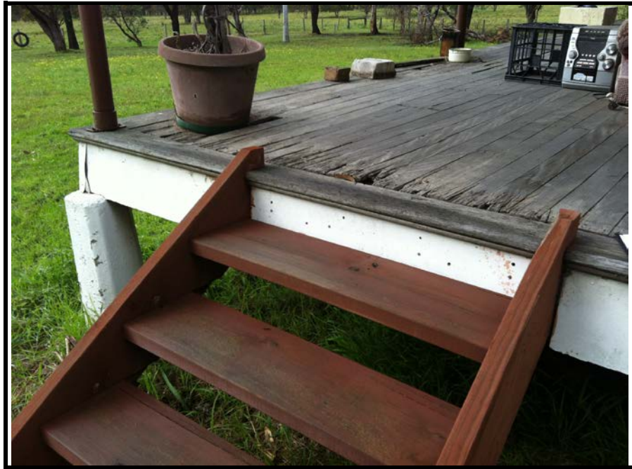
Photo 5: A section of the panels that are around the base of the verandah on the back and southern side of the house. Laboratory analysis concluded these are not ACM.
