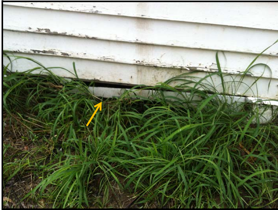
Photo 9: One of the sections of ACM sheeting used as infill panels between the house and the ground on the western side of the house
