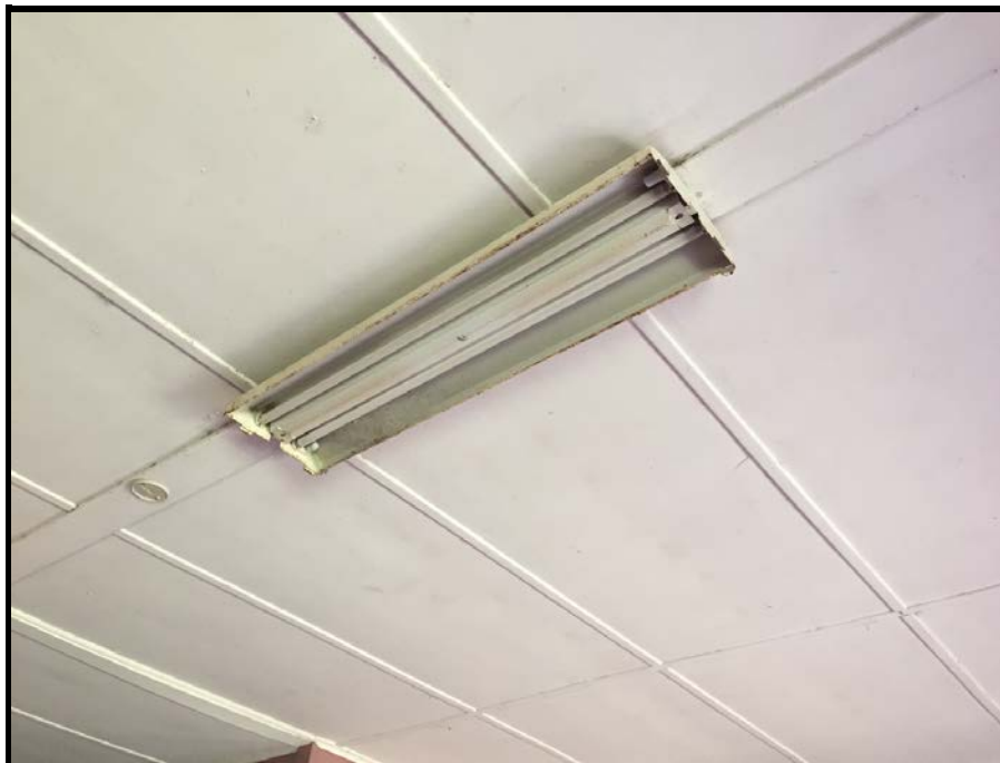
Photo 16: Fluorescent light fitting in the living area that potentially includes a PCB-containing capacitor.
