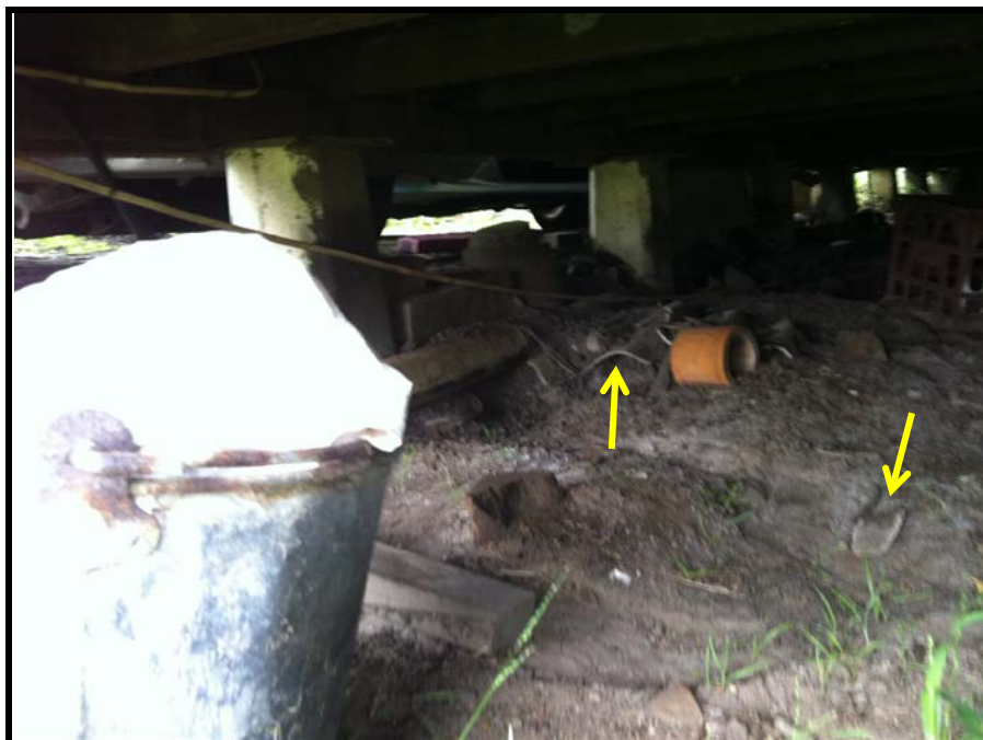
Photo 8: Arrows pointing to some of the fragments of corrugated ACM sheeting under the northwestern corner of the house
