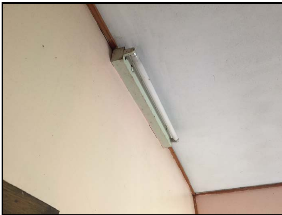
Photo 18: Fluorescent light fitting in to the laundry that potentially includes a PCB-containing capacitor.
