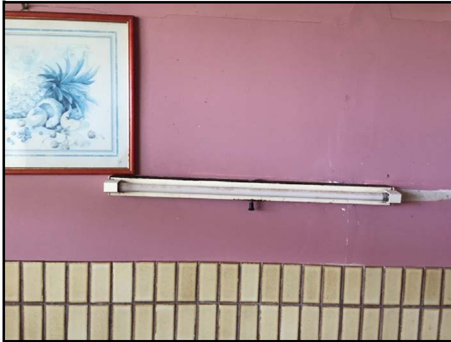
Photo 17: Fluorescent light fitting in to the kitchen wall that potentially includes a PCB-containing capacitor.
