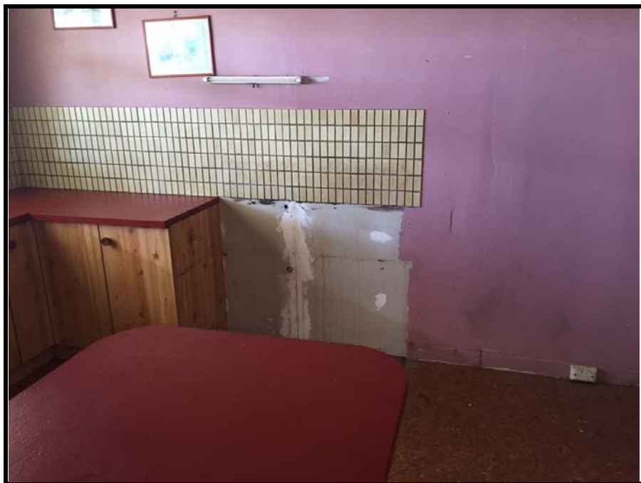
Photo 14: Section of the ACM wall in the kitchen area.
