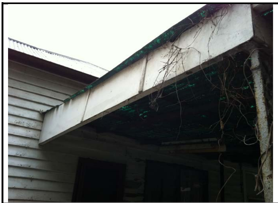
Photo 2: Part of the ACM panelling around the top of the carport.
