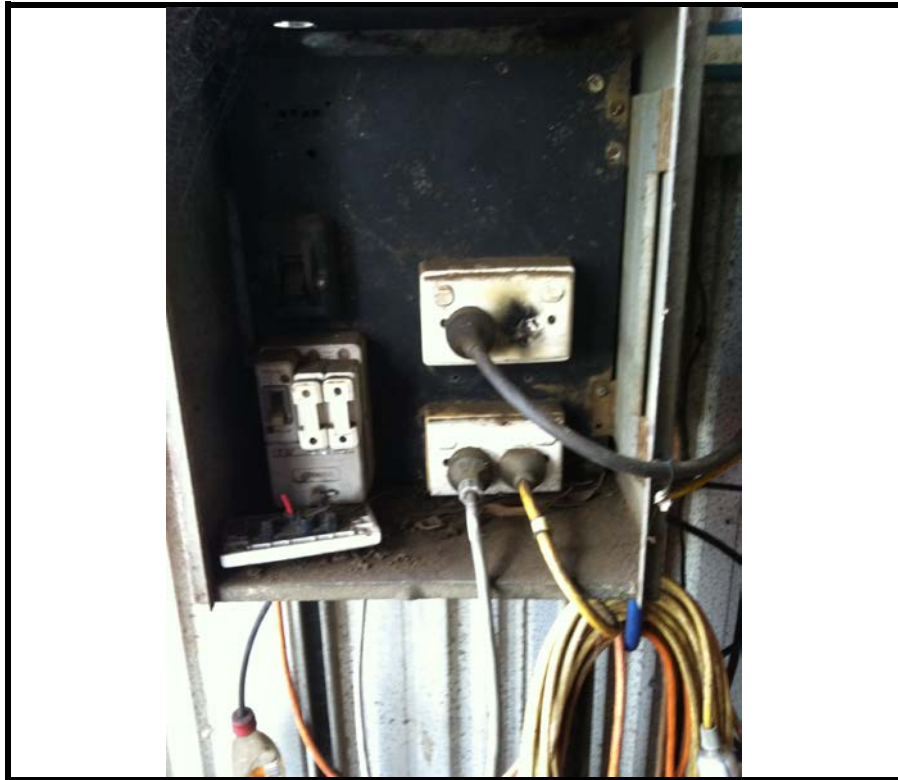
Photo 11: The electrical power box in the garage with a zelemite backing board.
