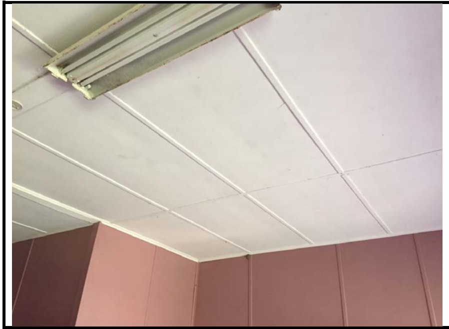
Photo 15: Section of the ACM lined ceiling in the main section of the house.
